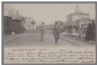
Lier, Station, Leopoldplein 34 (SLI001000622)
