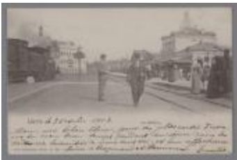
Lier, Station, Leopoldplein 34 (SLI001000622)
