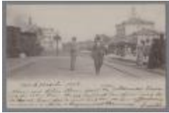
Lier, Station, Leopoldplein 34 (SLI001000622)
